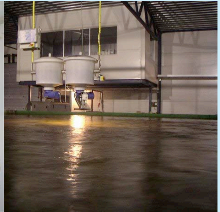
electrical spreader in Feeding Robot
